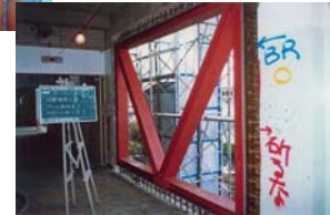
Retrofitting by steel brace
