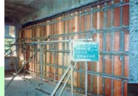
Replace brick wall to infill RC wall
